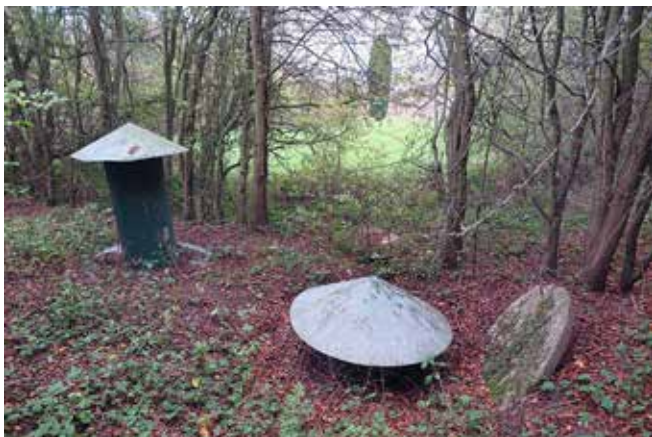
Welbeck Abbey: Ventilators above one of the tunnels. Photo Clive Penfold
